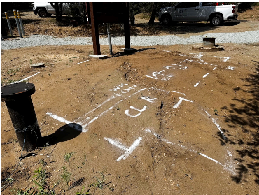
Well 14 Pump Station Building layout marked by CWD staff.
